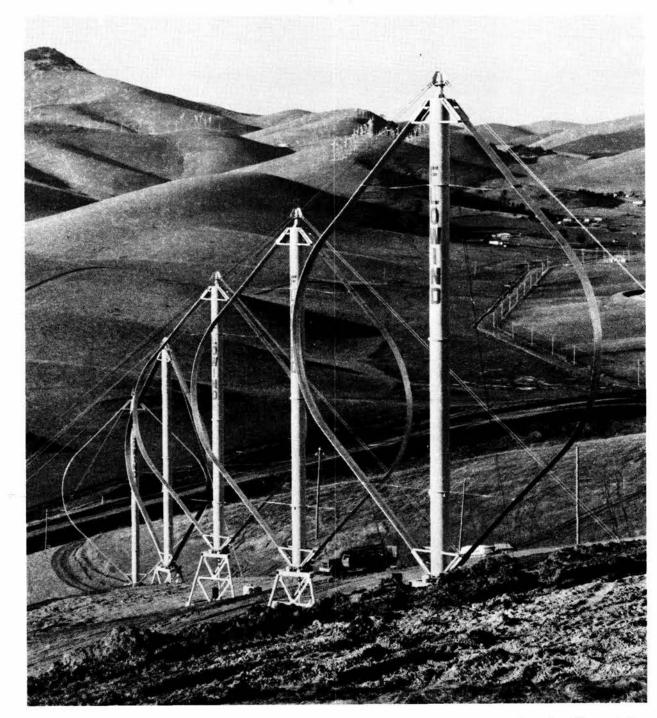
WHAT VAWT HATH WROUGHT — Rows of vertical axis wind turbines can be seen along the Altamont Pass off Interstate 580 these days as the FloWind Corporation of Kent, Wash. erects the 92-foot-tall windmills to harness the abundant wind energy blowing through the hills. This model can produce 170 kW peak power. FloWind plans to install 400 machines this year east of Livermore. (Photo by Dick Jones, 8441)
